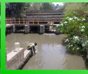
DELHI GATE DRAIN
