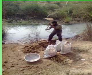
MORI GATE DRAIN
