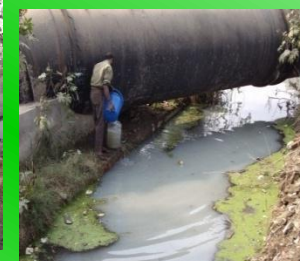
KHYBER PASS DRAIN
