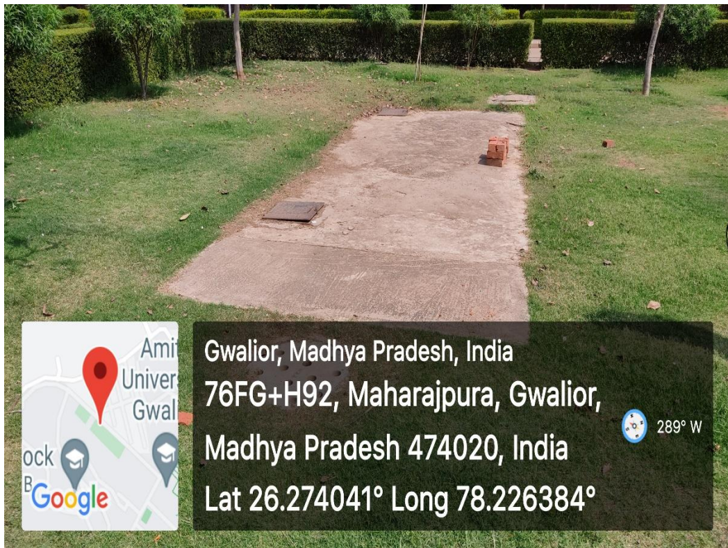
Rain Water Harvesting System
