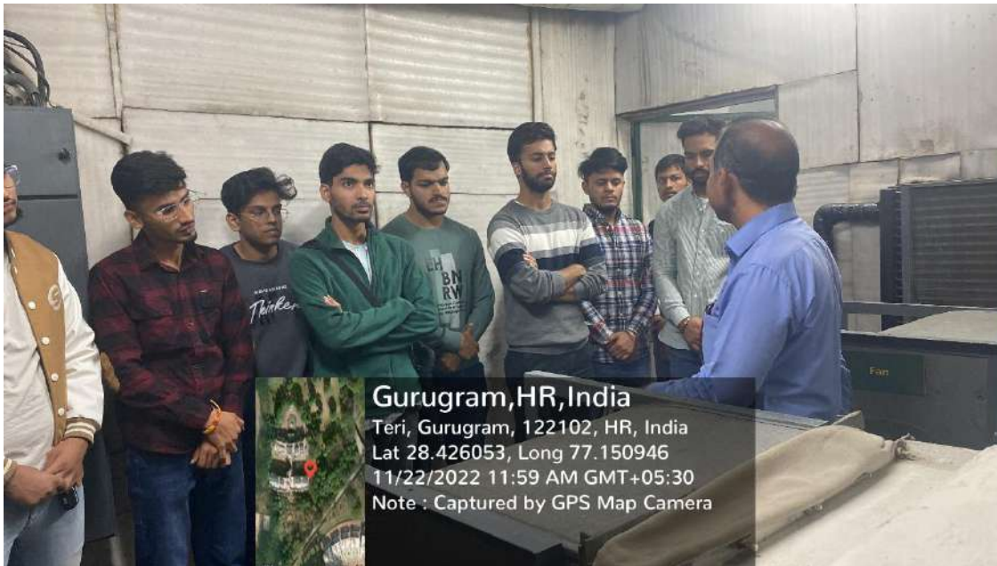
Fig. Fan room ( underground tunnel + dehumidifier) for air circulation ( heating & cooling)
