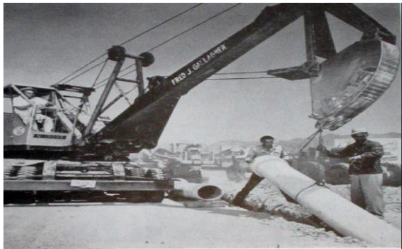
Fig. 2. Concrete pipe handling using crowbar
