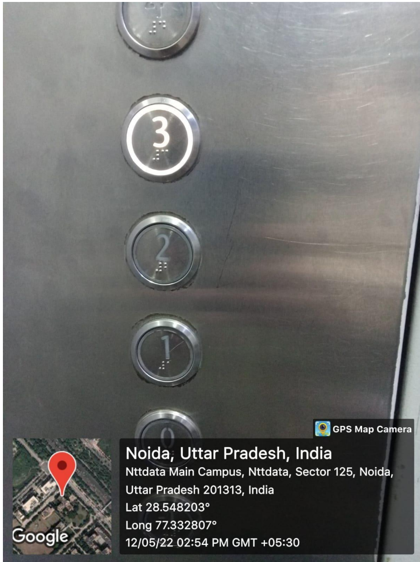
Figure 7.1.7.7: Braille enabled lift labels
